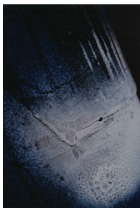
Fig. 1. Cracks in fillet welds
