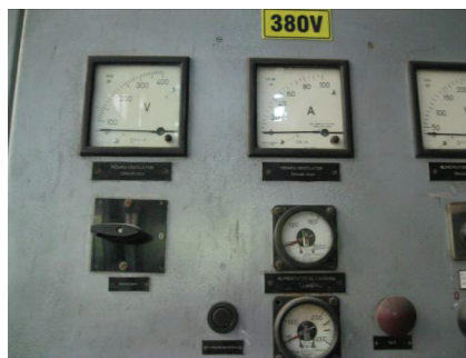
Fig.7. Measurement of electrical parameters of coal mill
