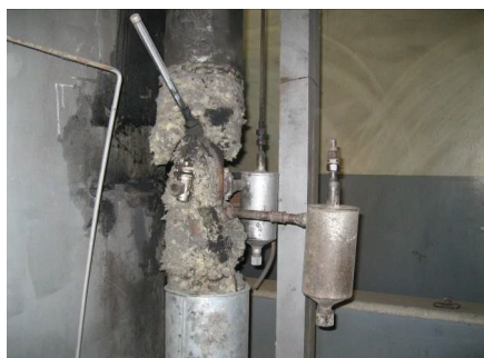
Fig.6. The system for coal dust capture located on the burner supply line
