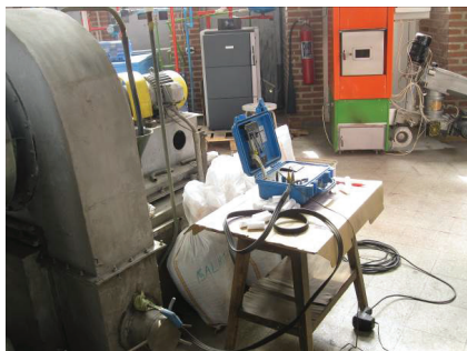
Fig.9. The location of the NO x measurement point at the end of the system (after the flue gas fan)
