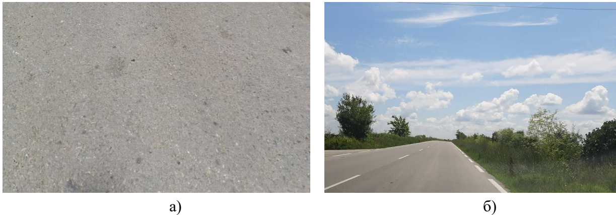
Fig. 3. General view of fine-grained surface: a - flat fine-grained surface; b - experimental section
