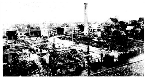
Fig. 1.2 Shoe factory after the boiler explosion of March 20, 1905 which led to the adoption of many state boiler codes and the ASME Boiler and Pressure Vessel Code. (Courtesy of Hartford Steam Boiler Inspection & Insurance Company)
