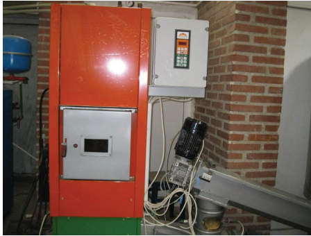
Figure 1. The ERPEK boiler of 40 kW
