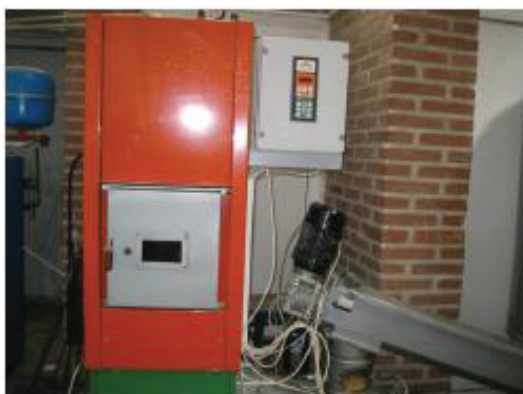
Figure 7. 40 kW ERPEK boiler
