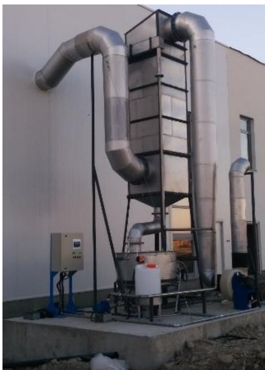
Fig. 4 Shows an existing acid gas cleaning installation
