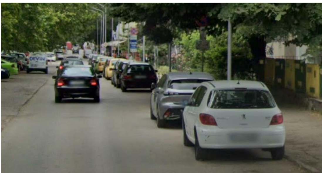
Fig. 3 Lack of markings and safety barriers
