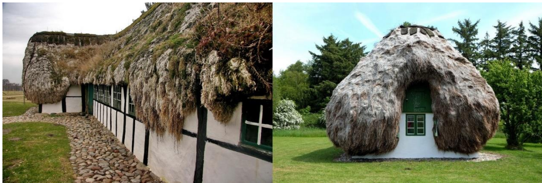
Fig. 2. Traditional roofs made of seaweed on the island of Læsø, Denmark. Photo sources: Gert Pedersen/Flickr; Jörg-Dieter Langhans/Flickr
